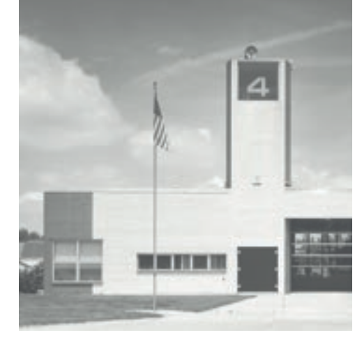
Fire Station No. 4, Venturi
